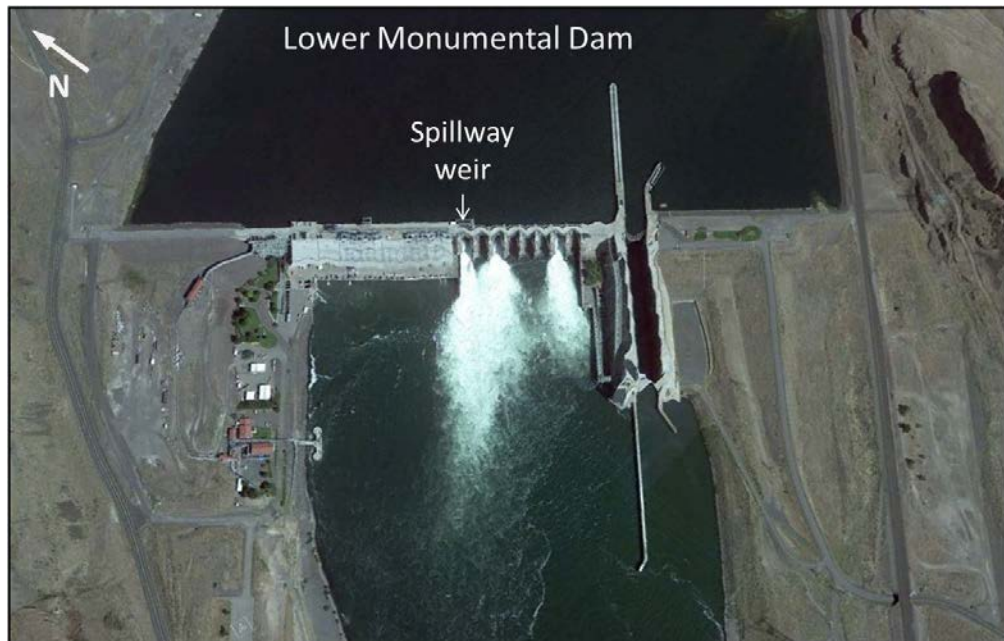
Figure 1.5. Aerial photograph of Lower Monumental Dam. The spillway weir (surface route) is located on the north side of the spillway.
